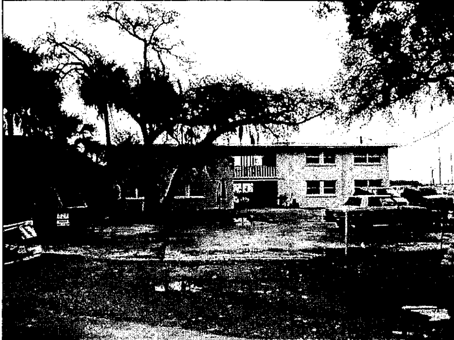
Multi-family building directly south of the main campus, Trout River Drive.
